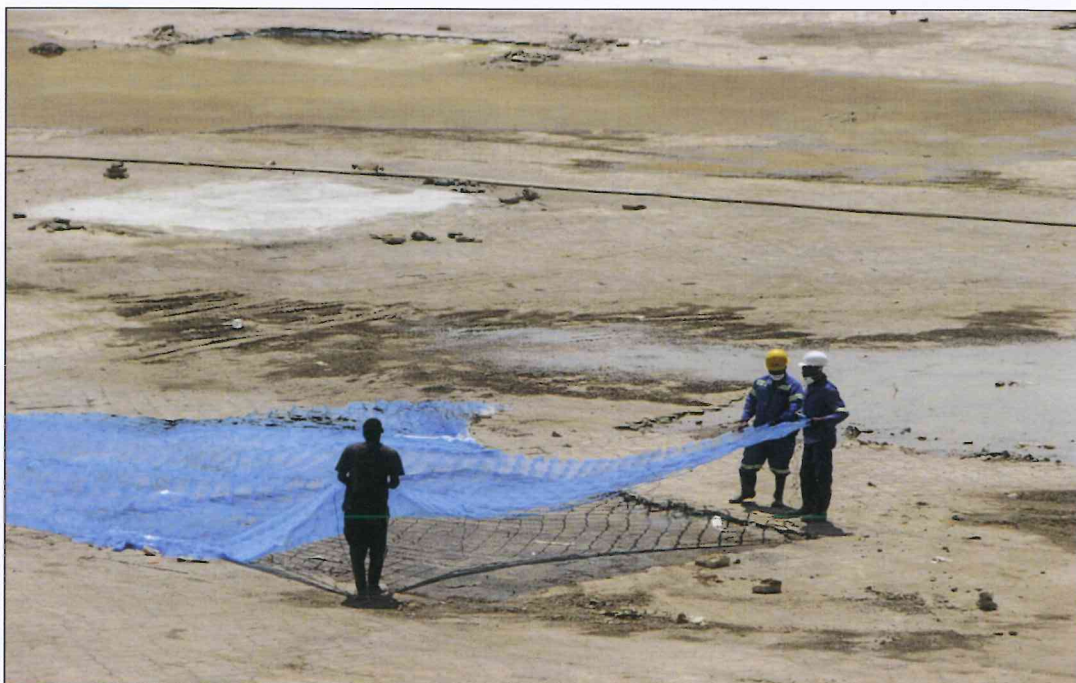
Repairs to the damaged floor of the Havercroft Reservoir.
