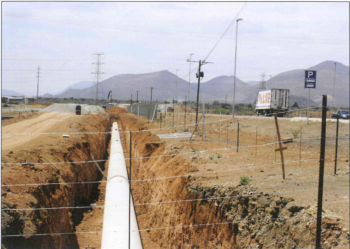
A portion of the Phase 2C Pipeline.
