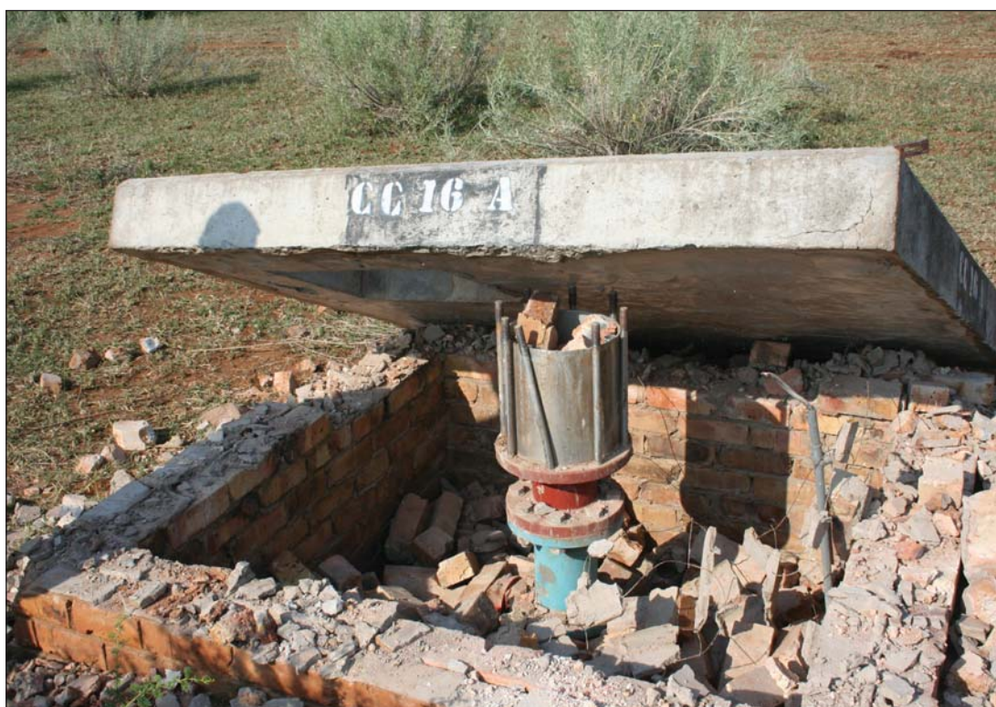
A vandalised air valve and chamber along the pipeline route.
