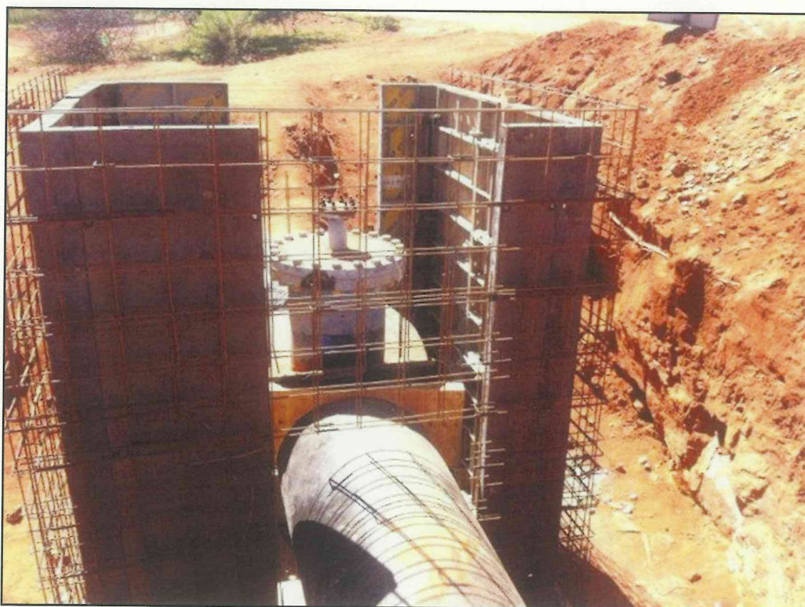
Reinforced concrete is now used for the housing of the valve chambers.
