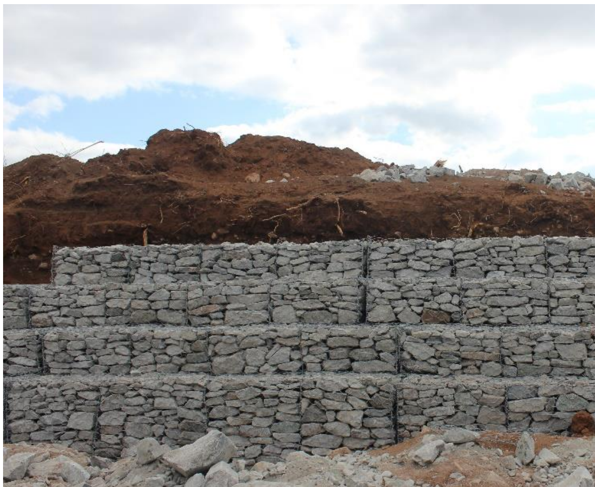
Photo 10: Clearance of vegetation found at the gabion embankment
