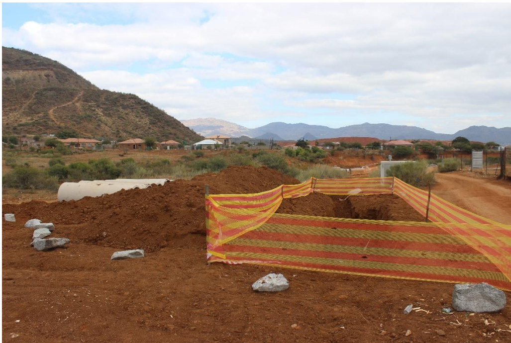
Photo 8: Topsoil stockpiled on site
