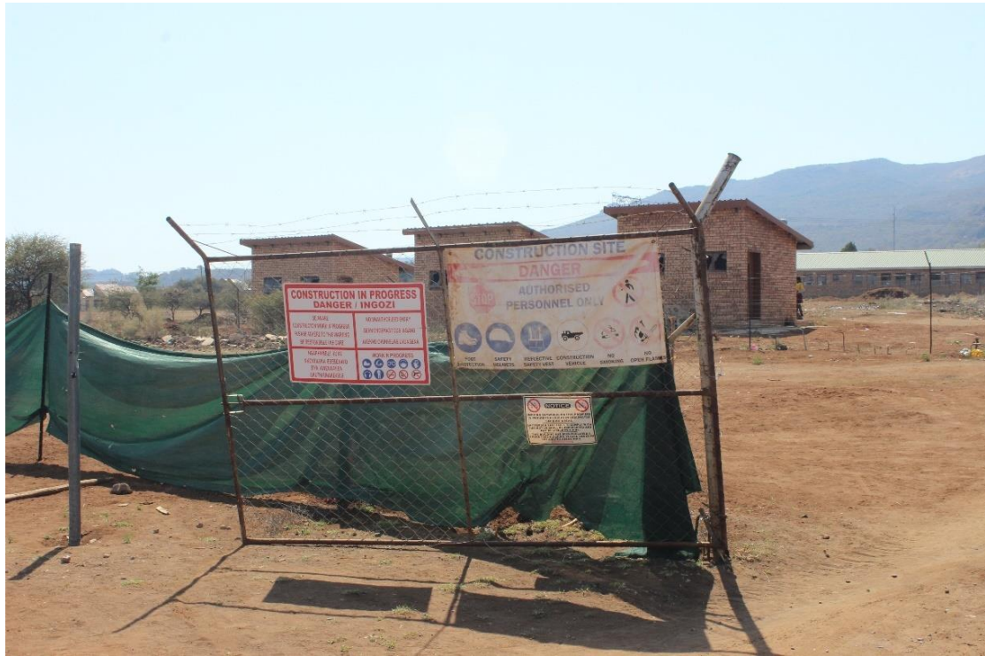
Photo 10: Laydown area and on-site offices within a fenced off area
