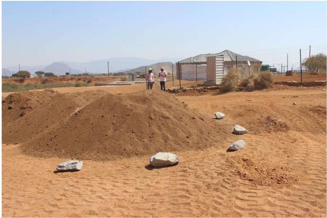
Photo 8: Topsoil stockpiled on site
