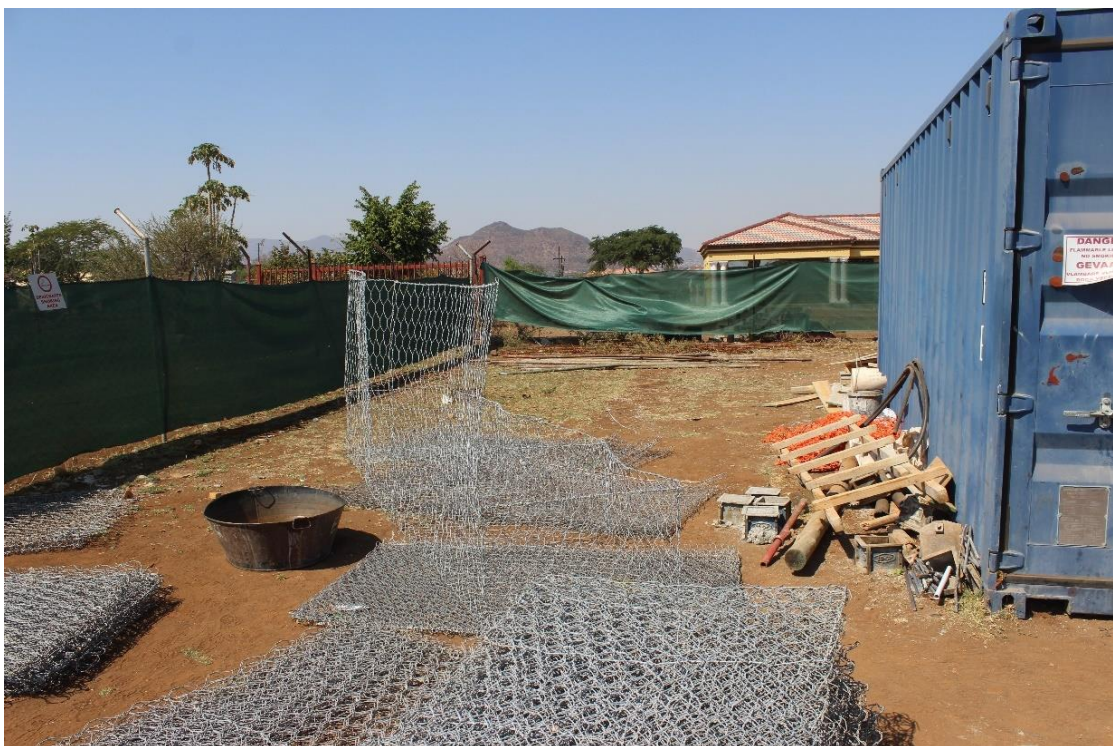
Photo 11: Laydown area and on-site offices within a fenced off area
