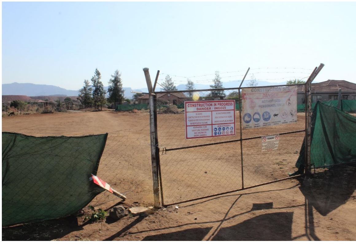
Photo 10: Laydown area and on-site offices within a fenced off area
