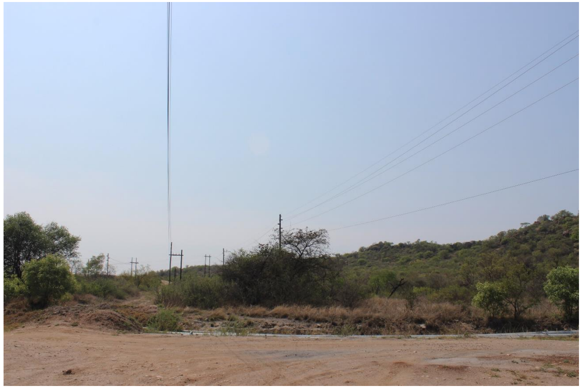
Photo 4: At Spitskop Pump Station
