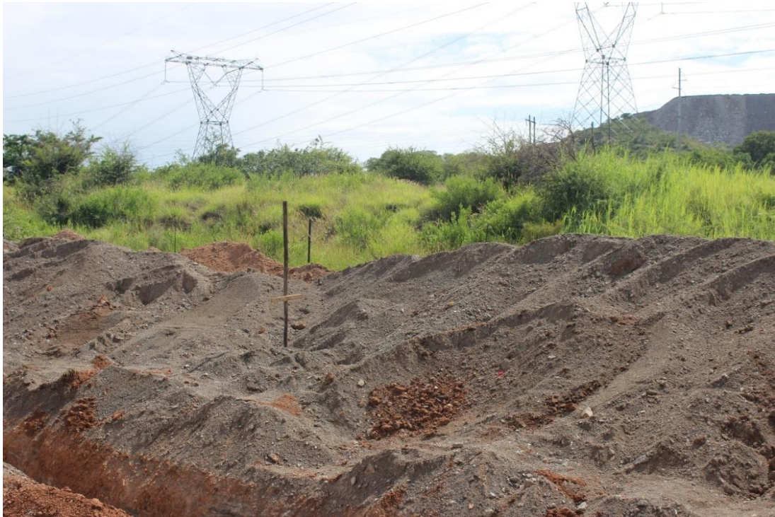
Photo 21: Separation of topsoil along pipeline
