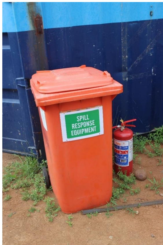
Photo 22: Hydrocarbon spill kit at the Spitskop Pump Station
