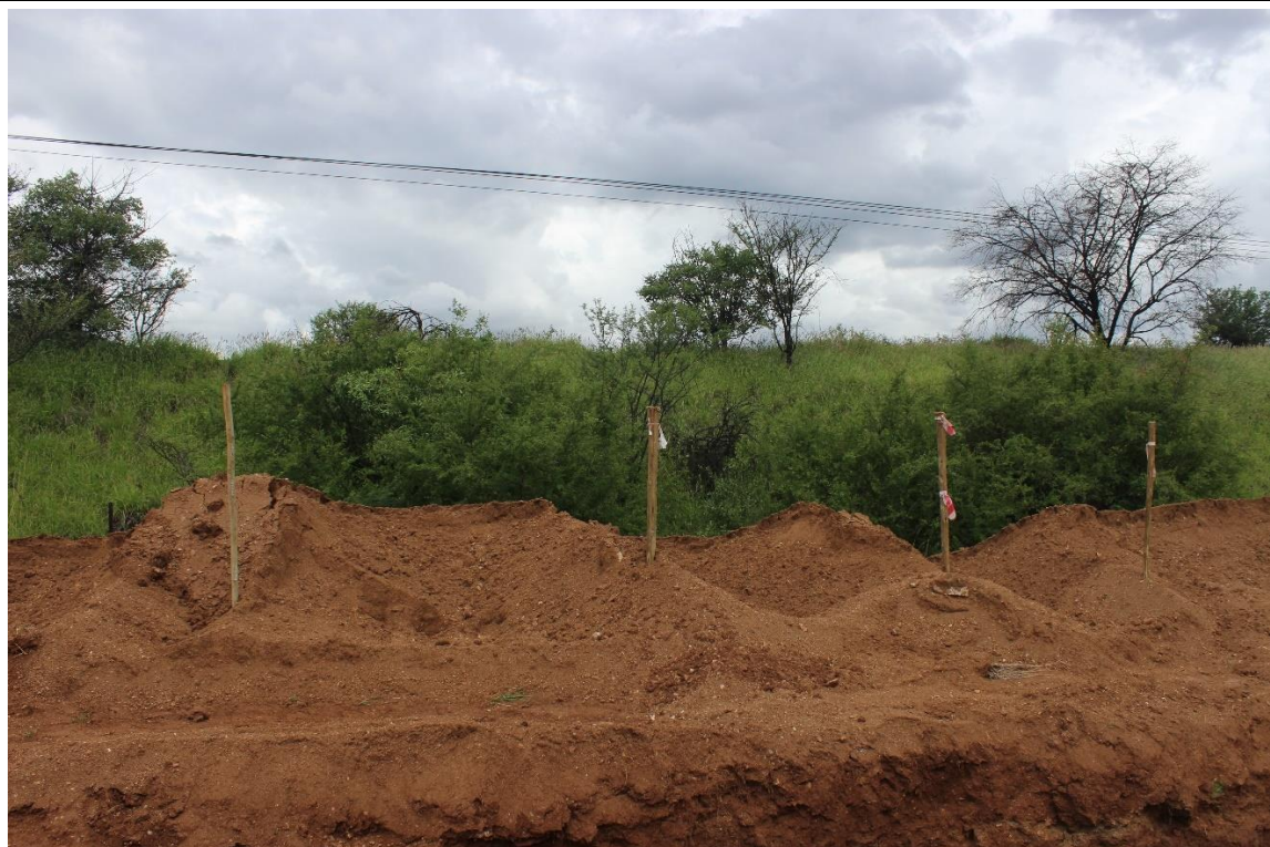
Photo 12: Micro-siting / pegging of the pipeline route
