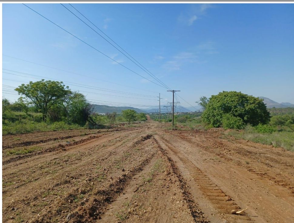
Photo 26: Clearance of vegetation along the pipeline route
