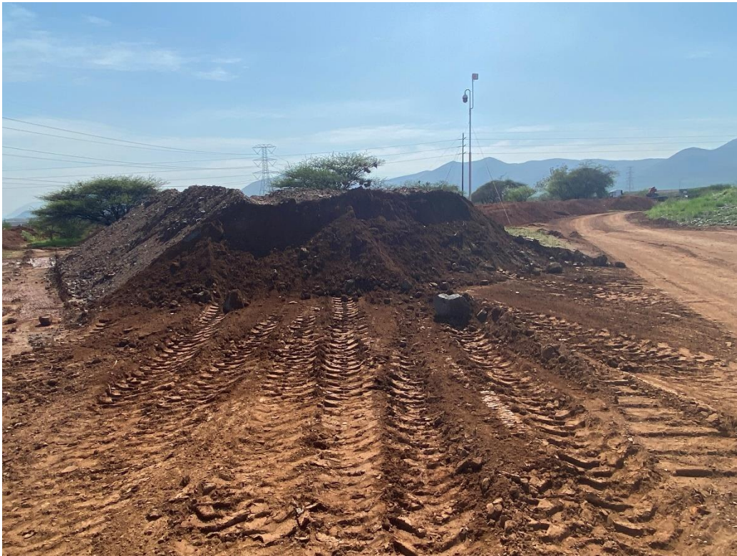
Photo 18: Separation of subsoil at the Spitskop Pump Station
