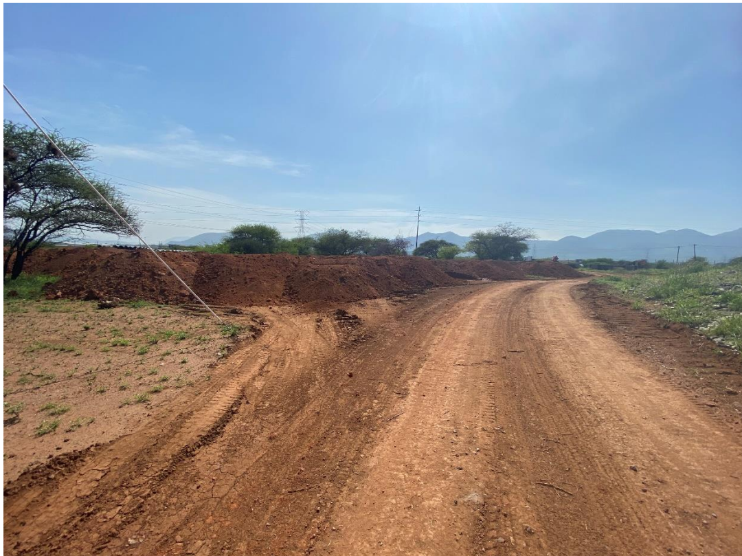
Photo 18: Separation of subsoil at the Spitskop Pump Station
