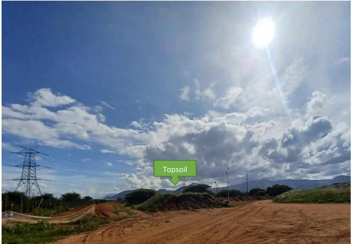
Photo 14: Stockpiles of topsoil on site.
