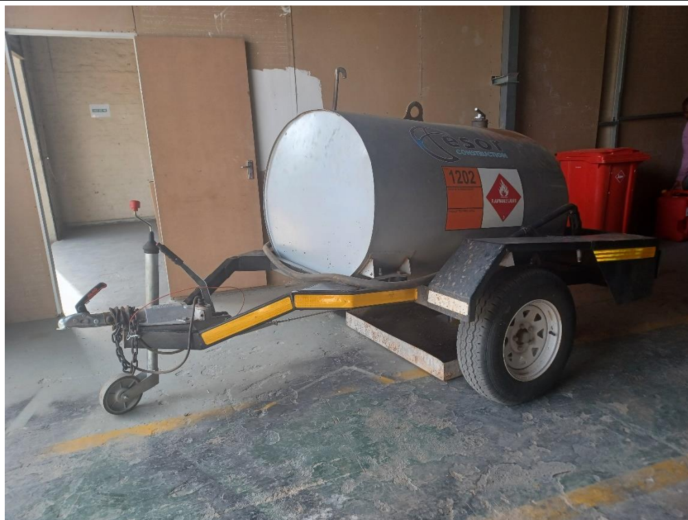
Photo 25: Drip trays under machinery not in use.
