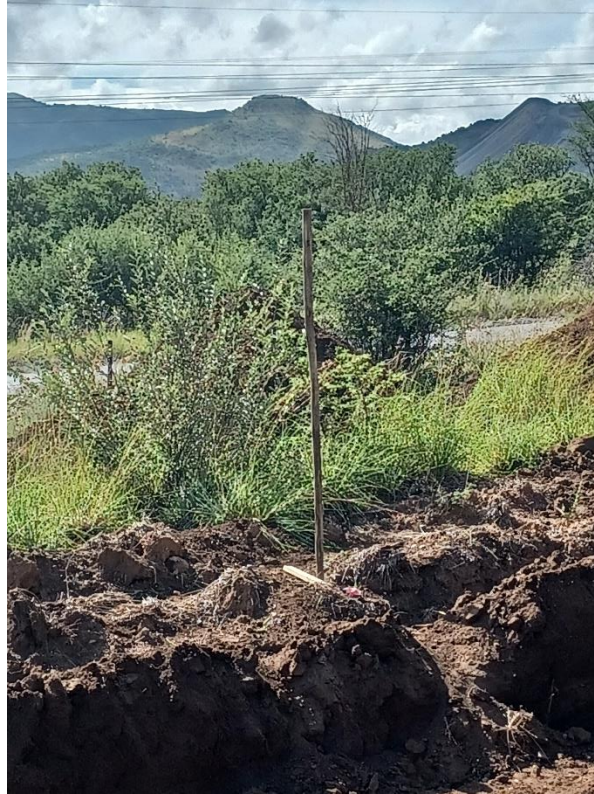
Photo 11: Micro-siting / pegging of the pipeline route
