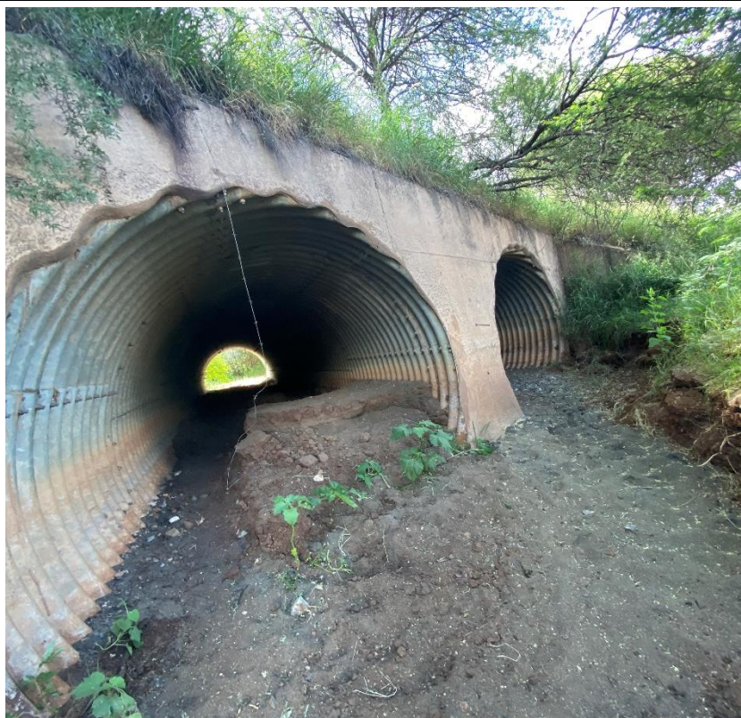
Photo 42: Drainage line culvert free from debris
