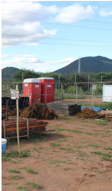
Photo 28: Ablution facility next to the pipeline
