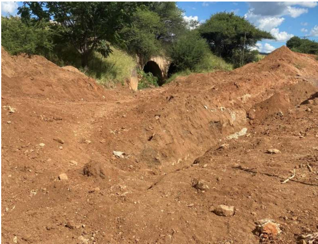
Photo 23: Soil stored in the drainageline and sandbags washed away
