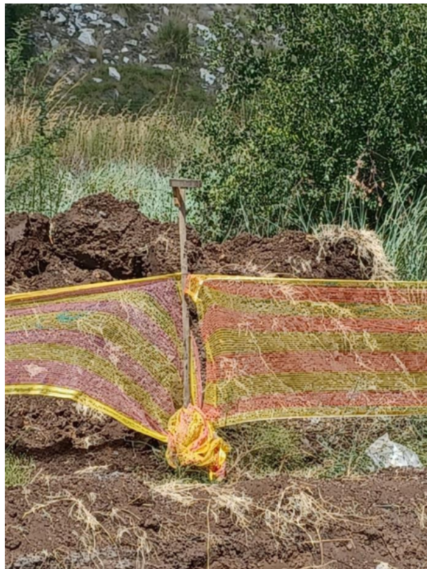
Photo 11: Micro-siting / pegging of the pipeline route
