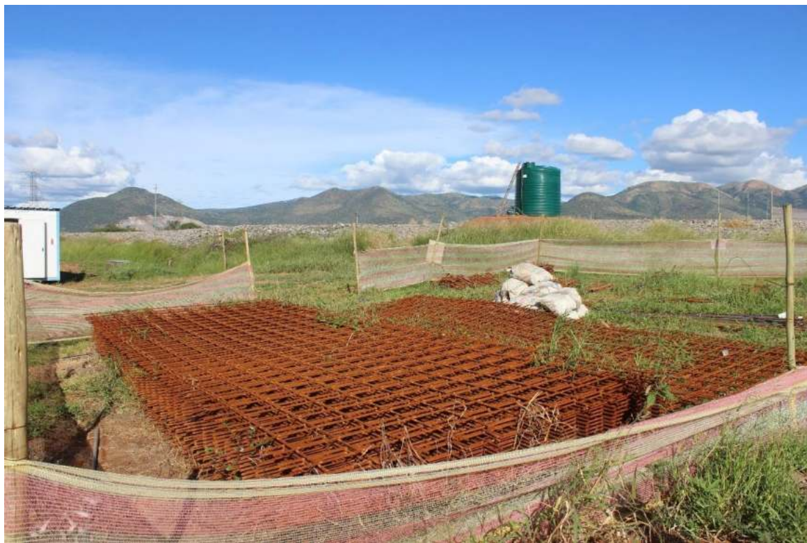
Photo 26: Construction footprint areas demarcated with reflector netting
