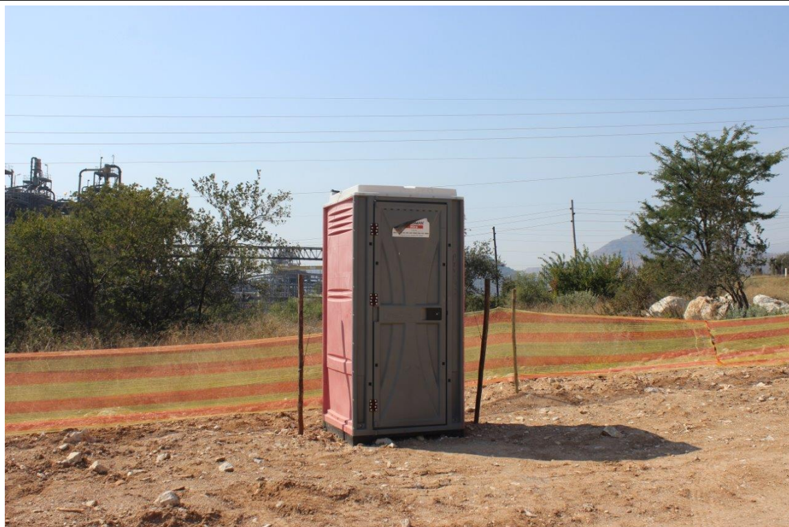
Photo 28: Ablution facility next to the pipeline
