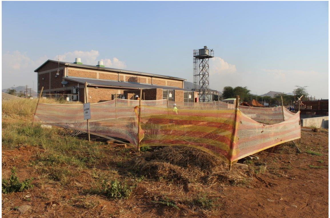
Photo 26: Construction footprint areas demarcated with reflector netting
