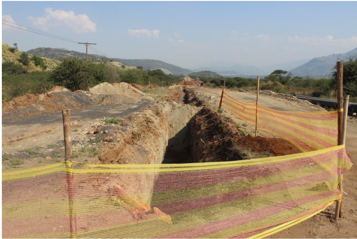
Photo 24: Construction activities within pipeline servitude
