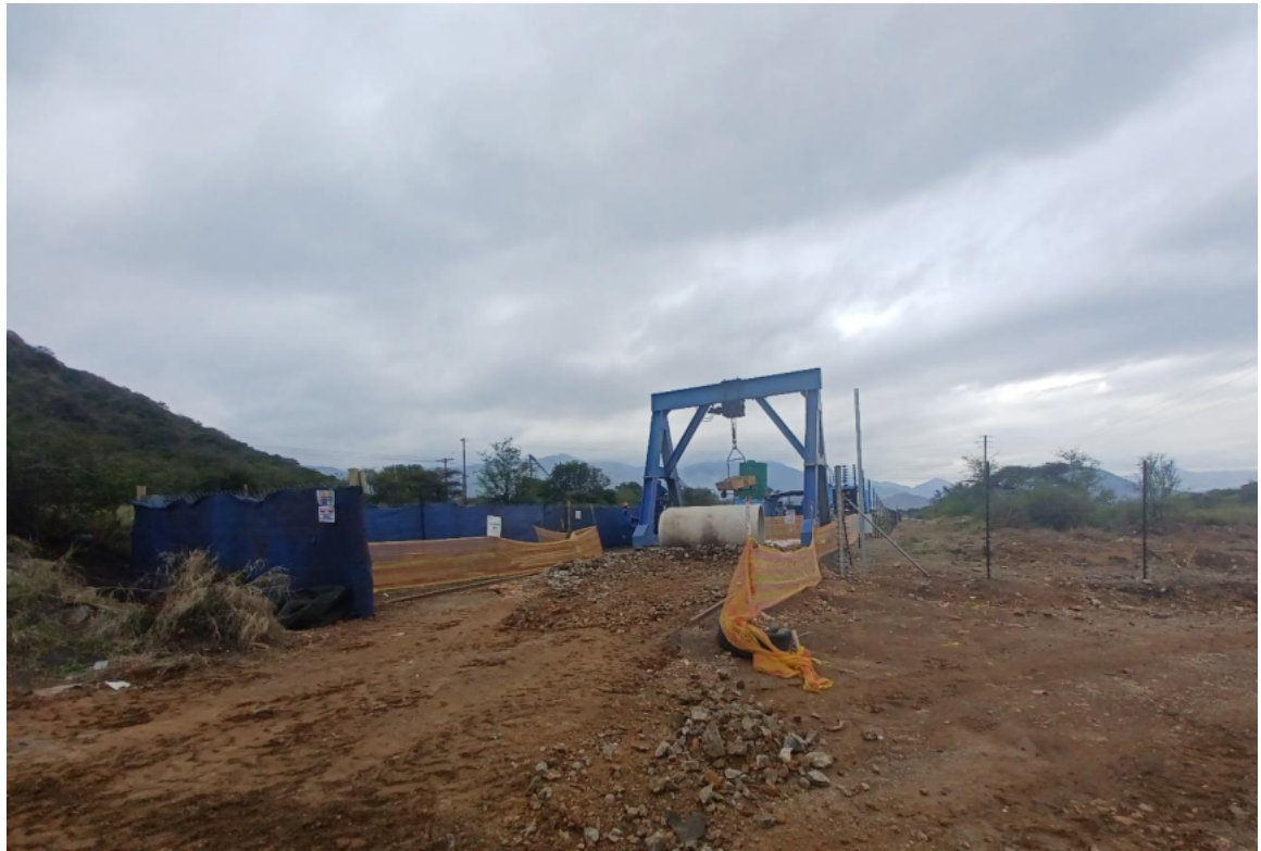
Photo 28: Construction footprint areas demarcated with reflector netting
