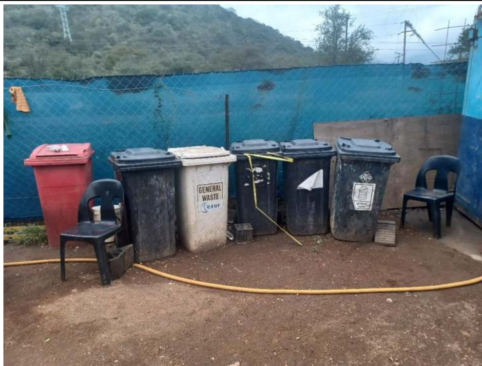
Photo 20: Waste Management on site (Pipe Jacking near Lion Smelter)
