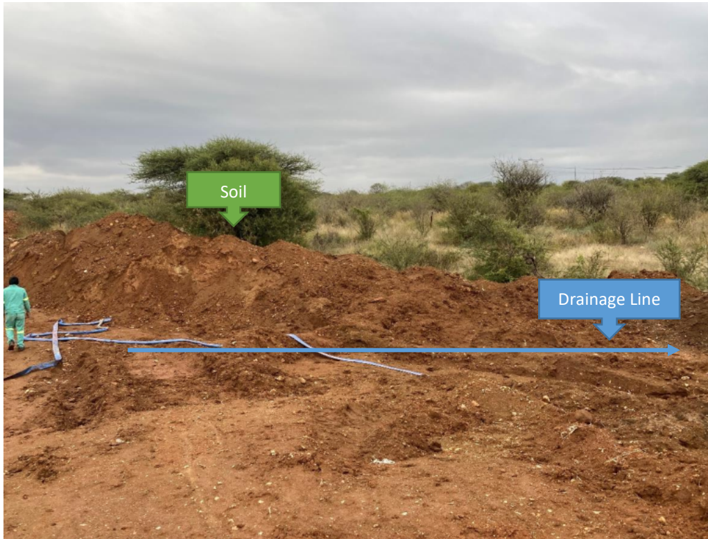
Photo 24: Soil stored in the drainageline and sandbags washed away
