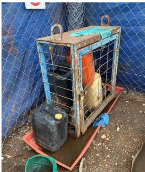
Photo 33: Correct Handling of Hazardous Chemical on site.
