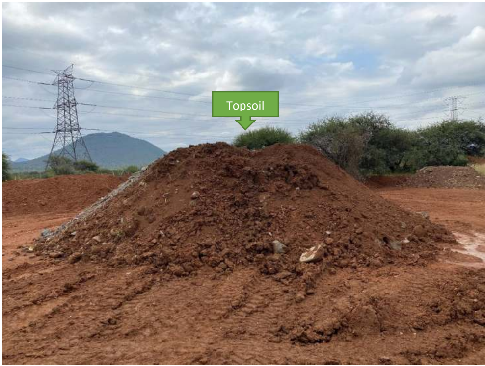
Photo 14: Stockpile of topsoil on site.
