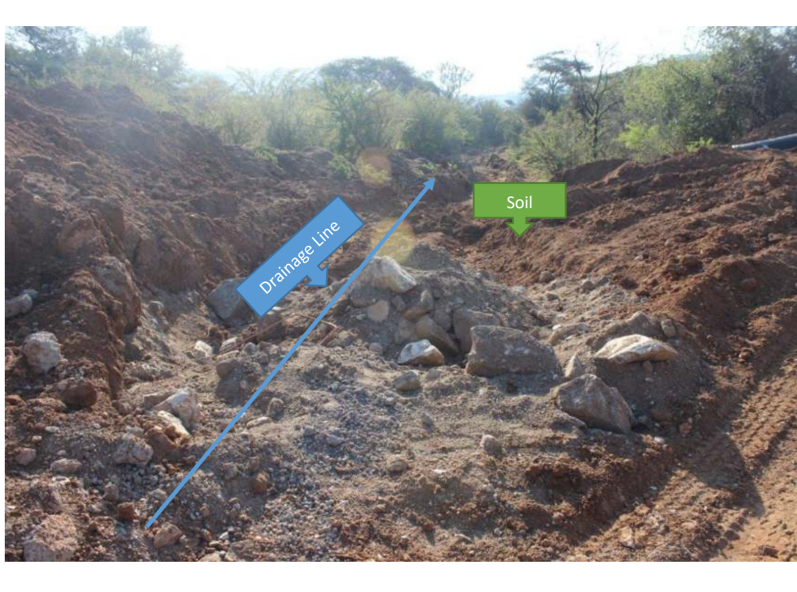
Photo 24: Soil stored in the drainageline and sandbags washed away
