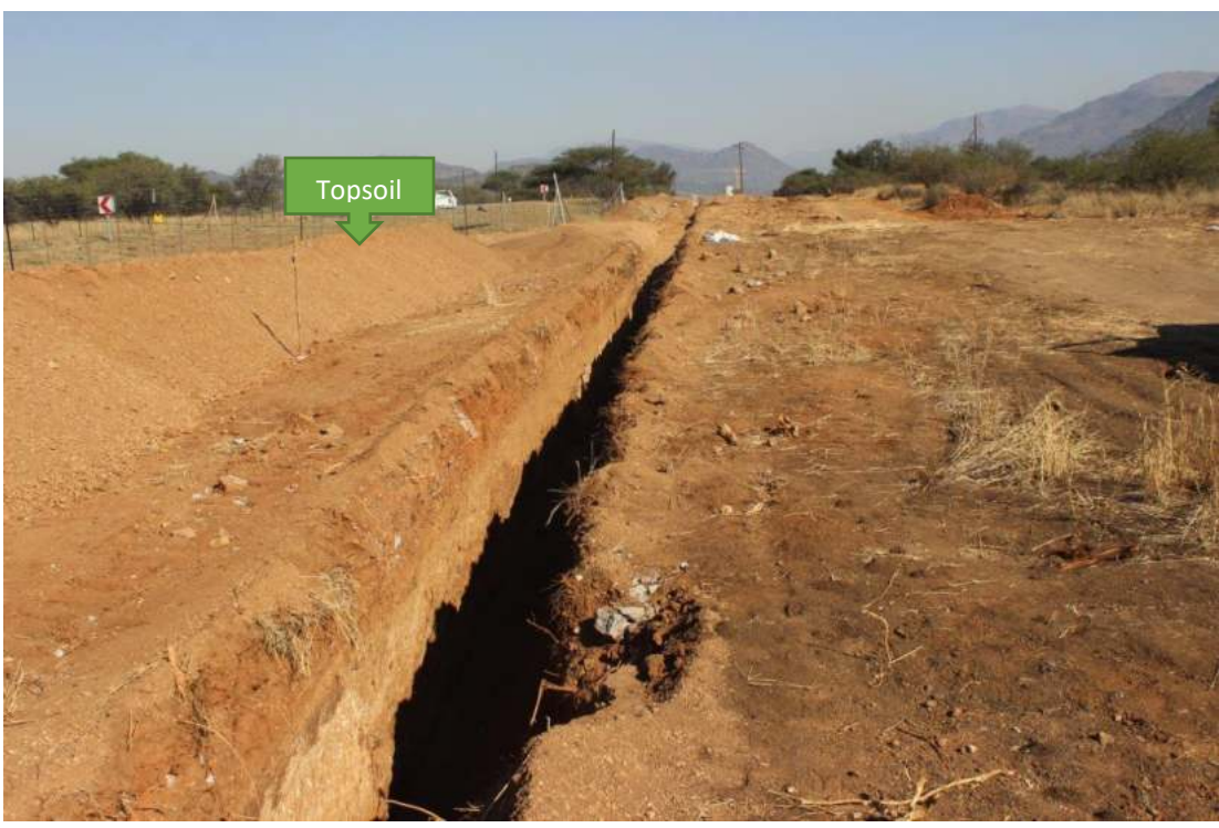
Photo 14: Stockpile of topsoil on site.
