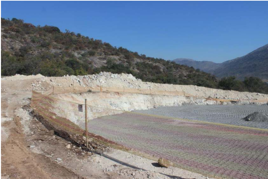
Photo 28: Construction footprint areas demarcated with reflector netting
