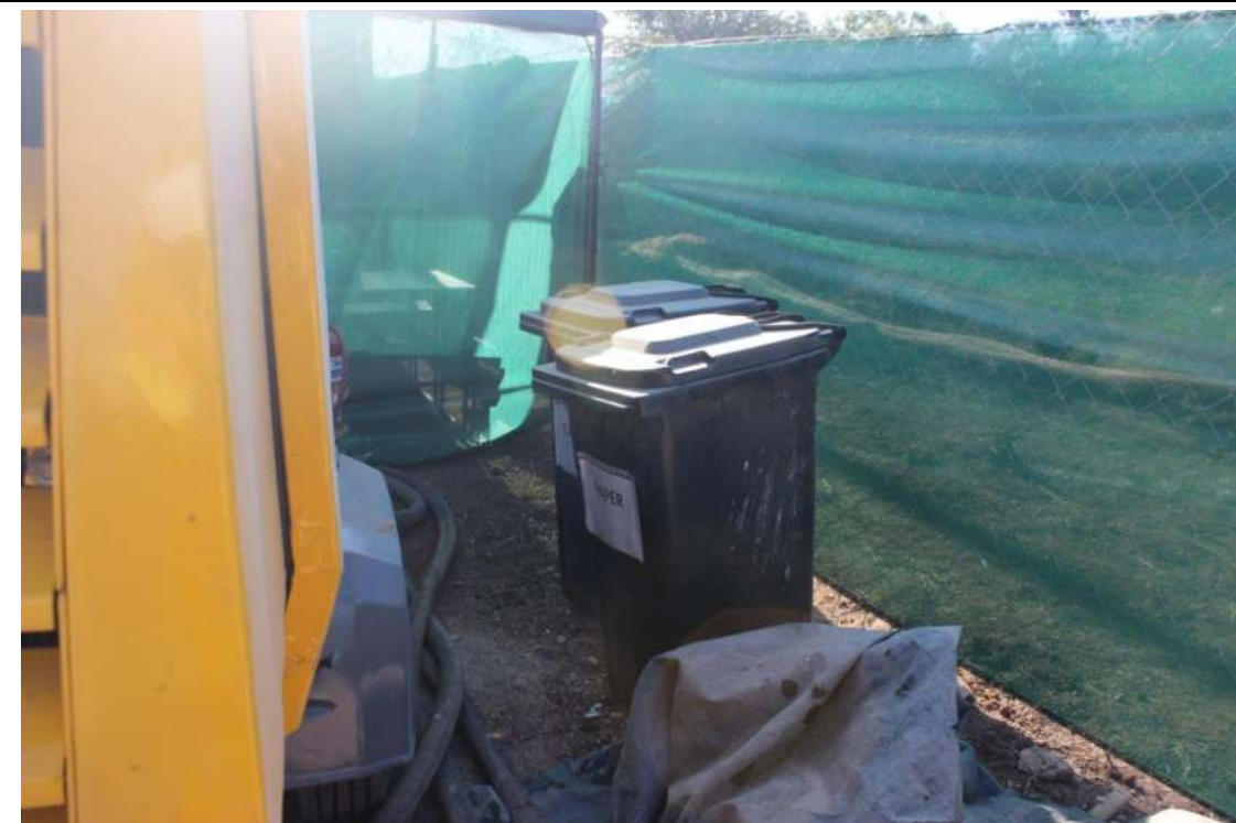
Photo 20: Waste Management on site (Pipe Jacking near Lion Smelter)
