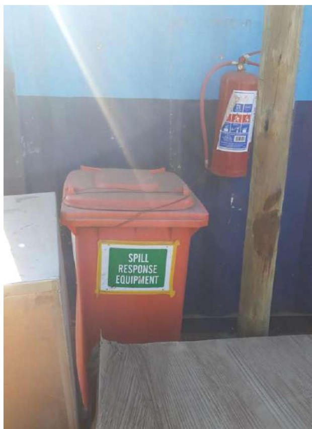
Photo 21: Hydrocarbon spill kits on site
