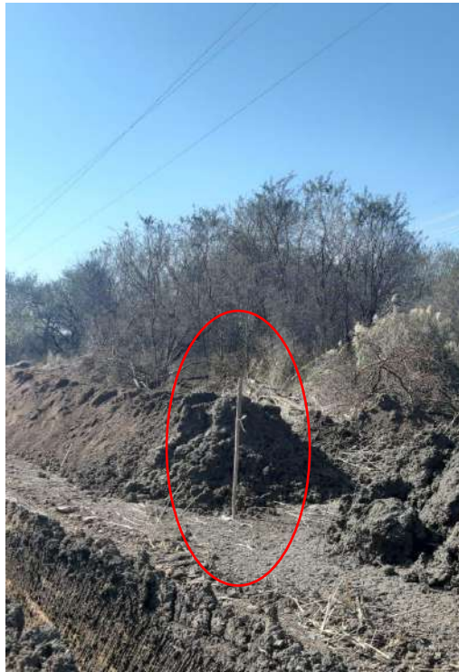
Photo 11: Micro-siting / pegging of the pipeline route
