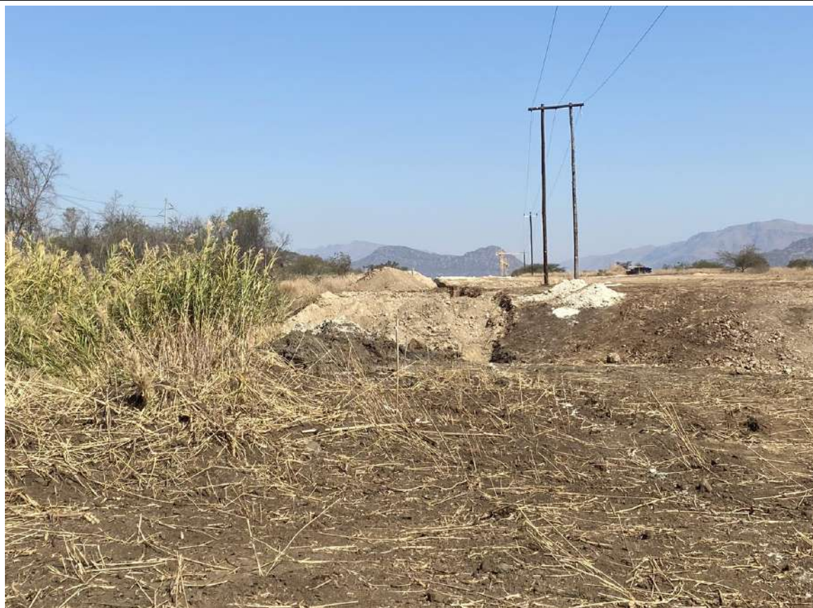
Photo 39: Wetland area – Construction activities undertaken
