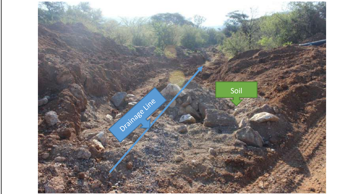
Photo 24: Soil stored in the drainageline and sandbags washed away
