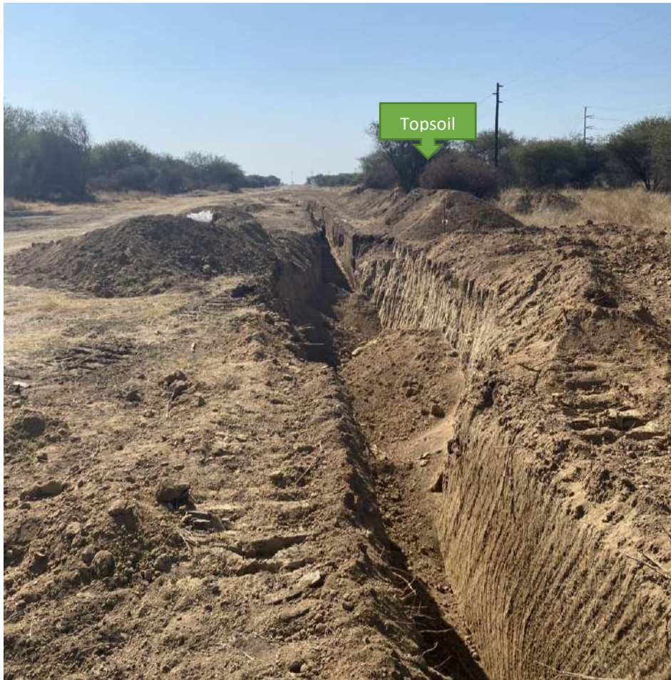
Photo 14: Stockpile of topsoil on site.
