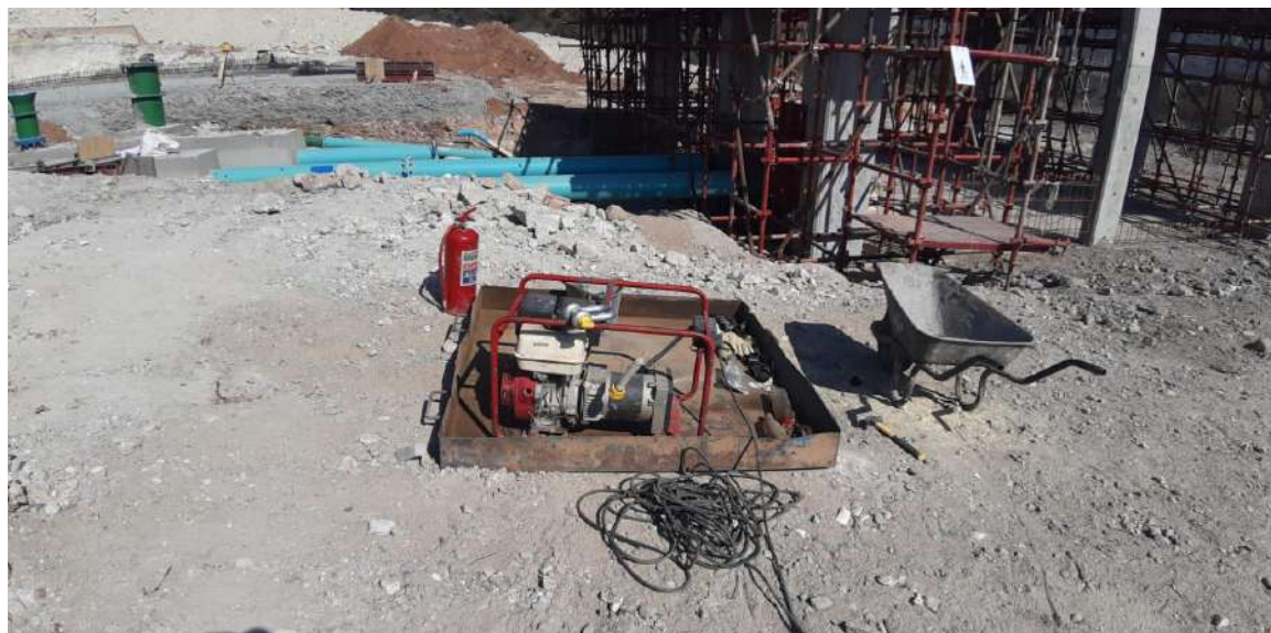
Photo 26: Drip trays under machinery not in use as well as no drip trays visible under machinery not in use.
