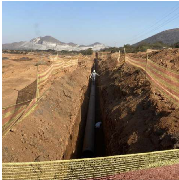
Photo 28: Construction footprint areas demarcated with reflector netting as well as construction areas not properly demarcated.
