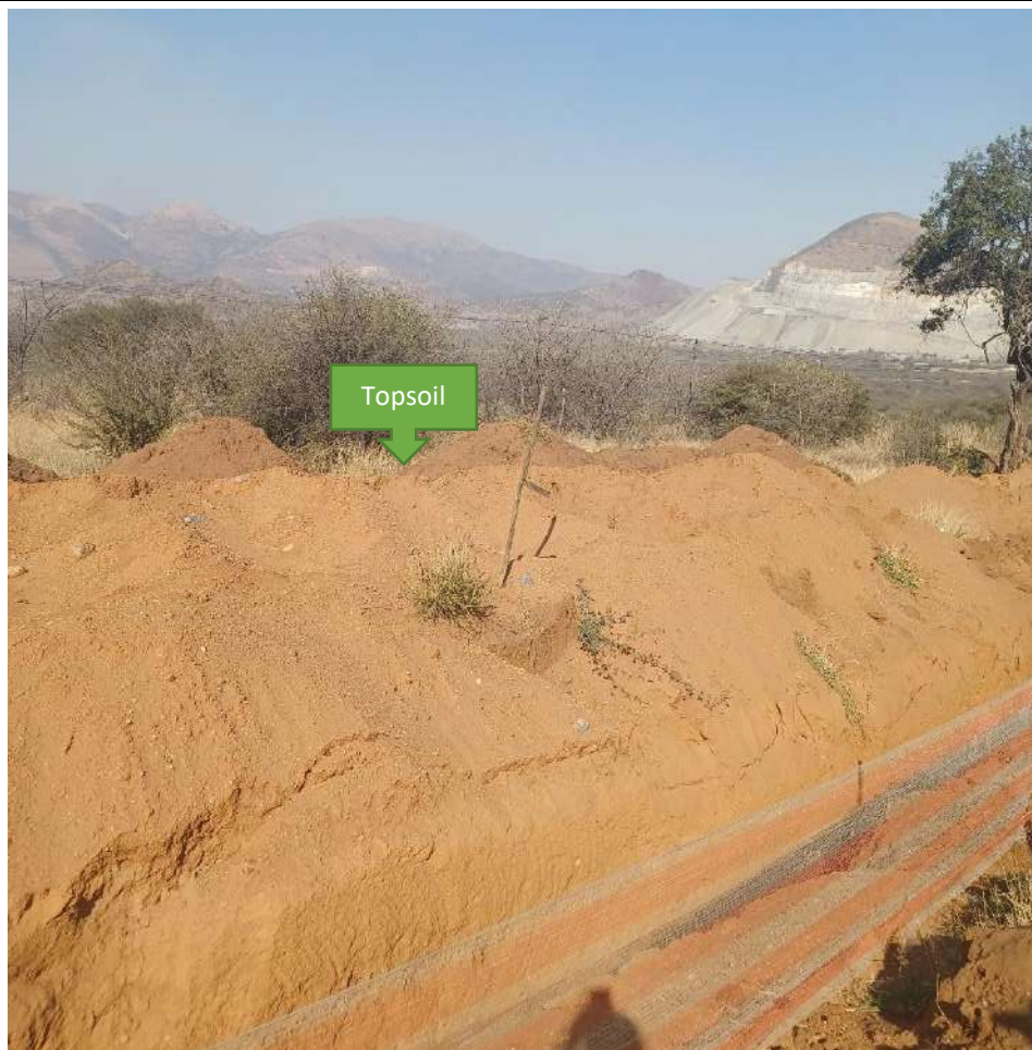
Photo 17: Stockpile of topsoil on site.
