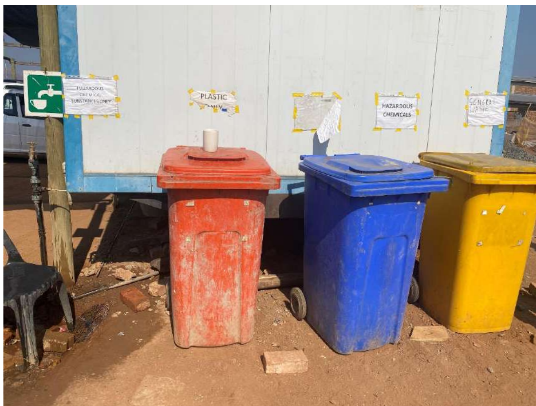
Photo 26: Spitskop Pump Station Waste Management
