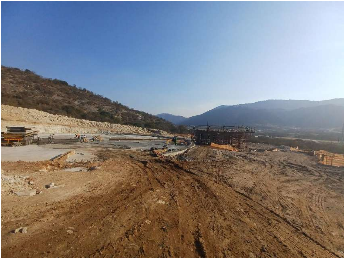
Photo 48: Deep hole excavation at Reservoir Site
