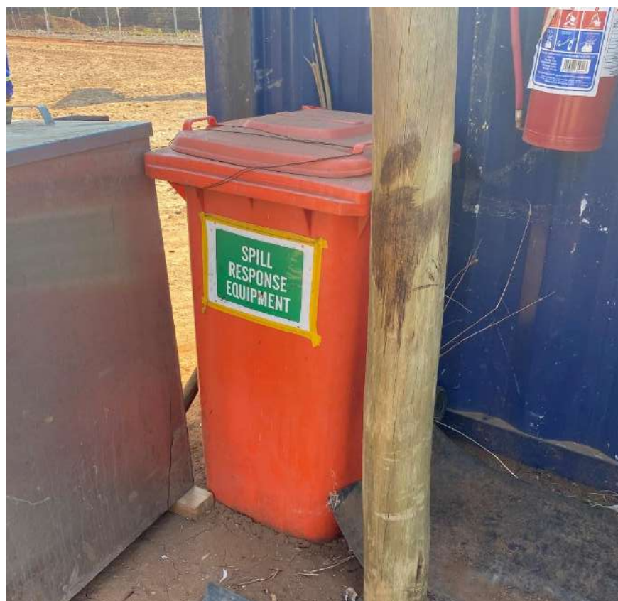
Photo 35: Hydrocarbon spill kits on site
