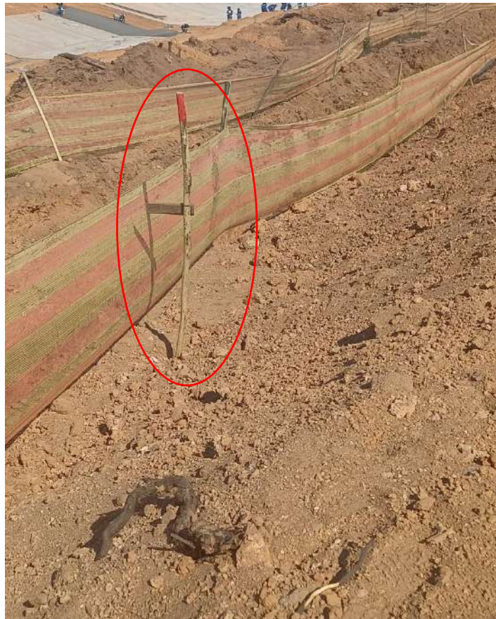
Photo 14: Micro-siting / pegging of the pipeline route
