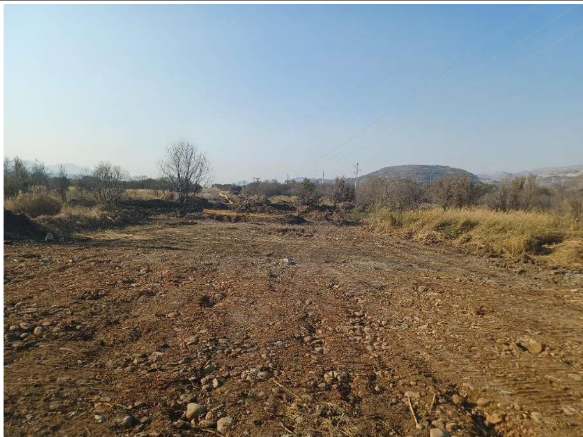
Photo 44: Wetland area – Construction activities undertaken
