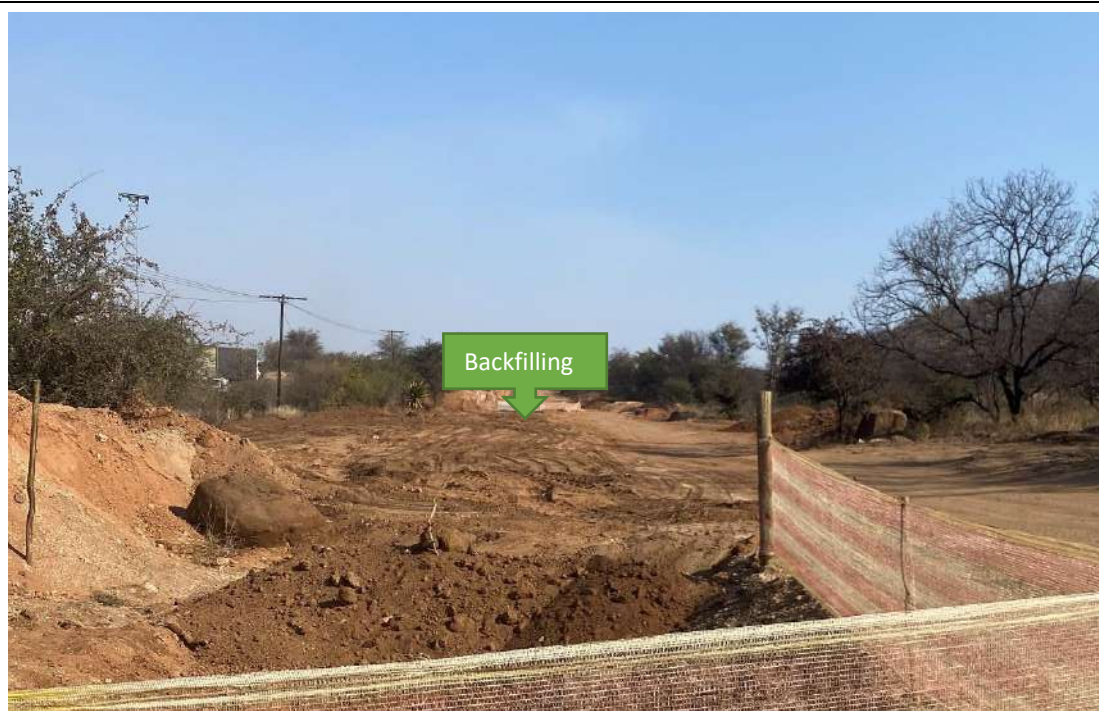
Photo 18: Backfilling of Subsoil on the pipeline route
