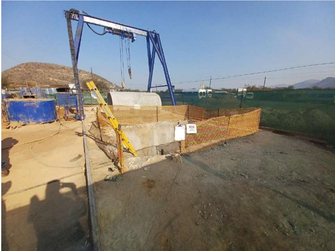
Photo 49: Deep hole excavation at Pipejacking Site
