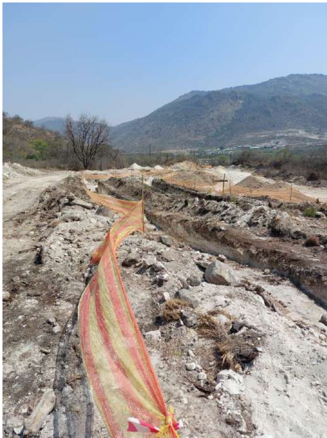
Photo 37: Construction footprint areas demarcated with reflector netting
