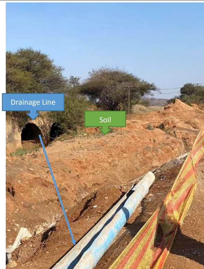
Photo 32: Soil stored in the drainageline and current construction activities
