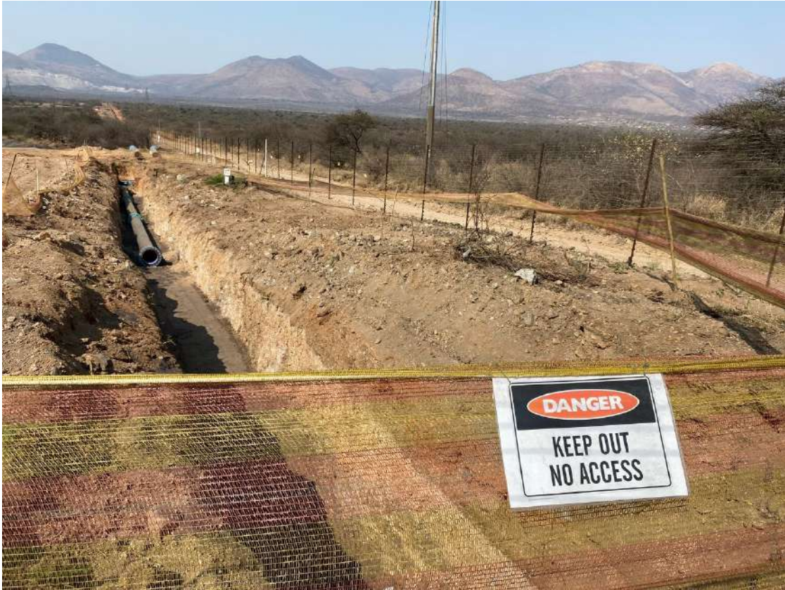
Photo 33: Construction activities within pipeline servitude
