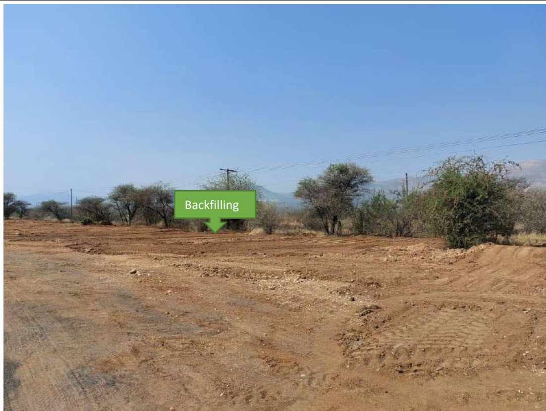
Photo 18: Backfilling of Subsoil on the pipeline route
