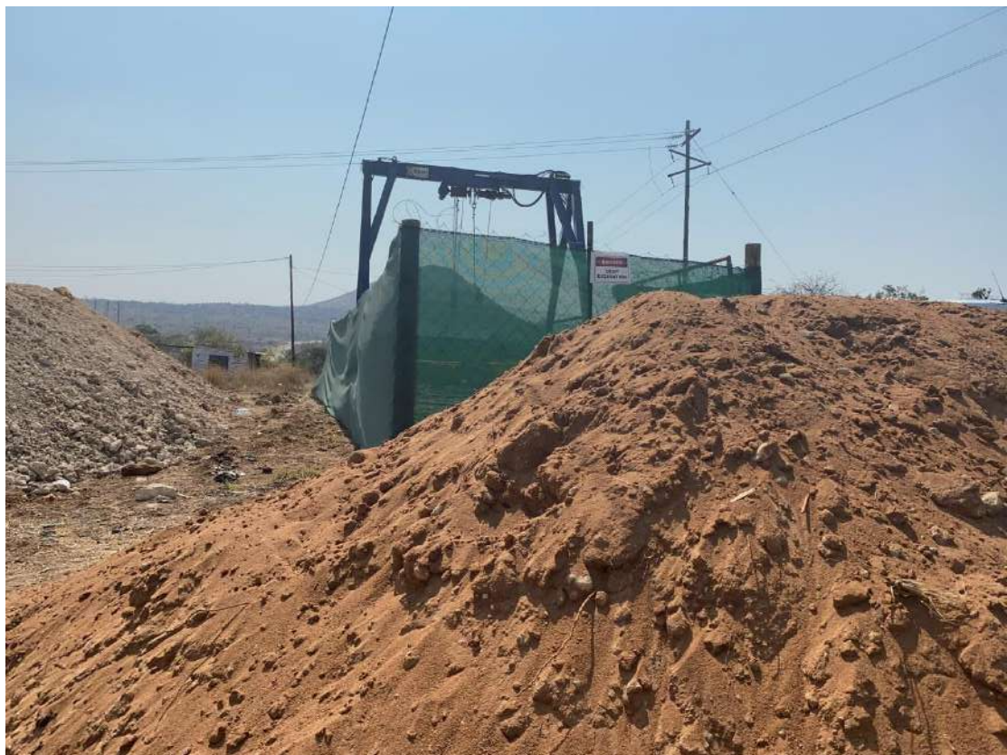
Photo 49: Deep hole excavation at Pipejacking Site
