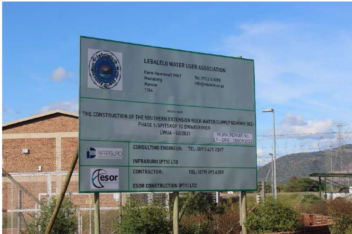
Photo 47: Construction signage on site
