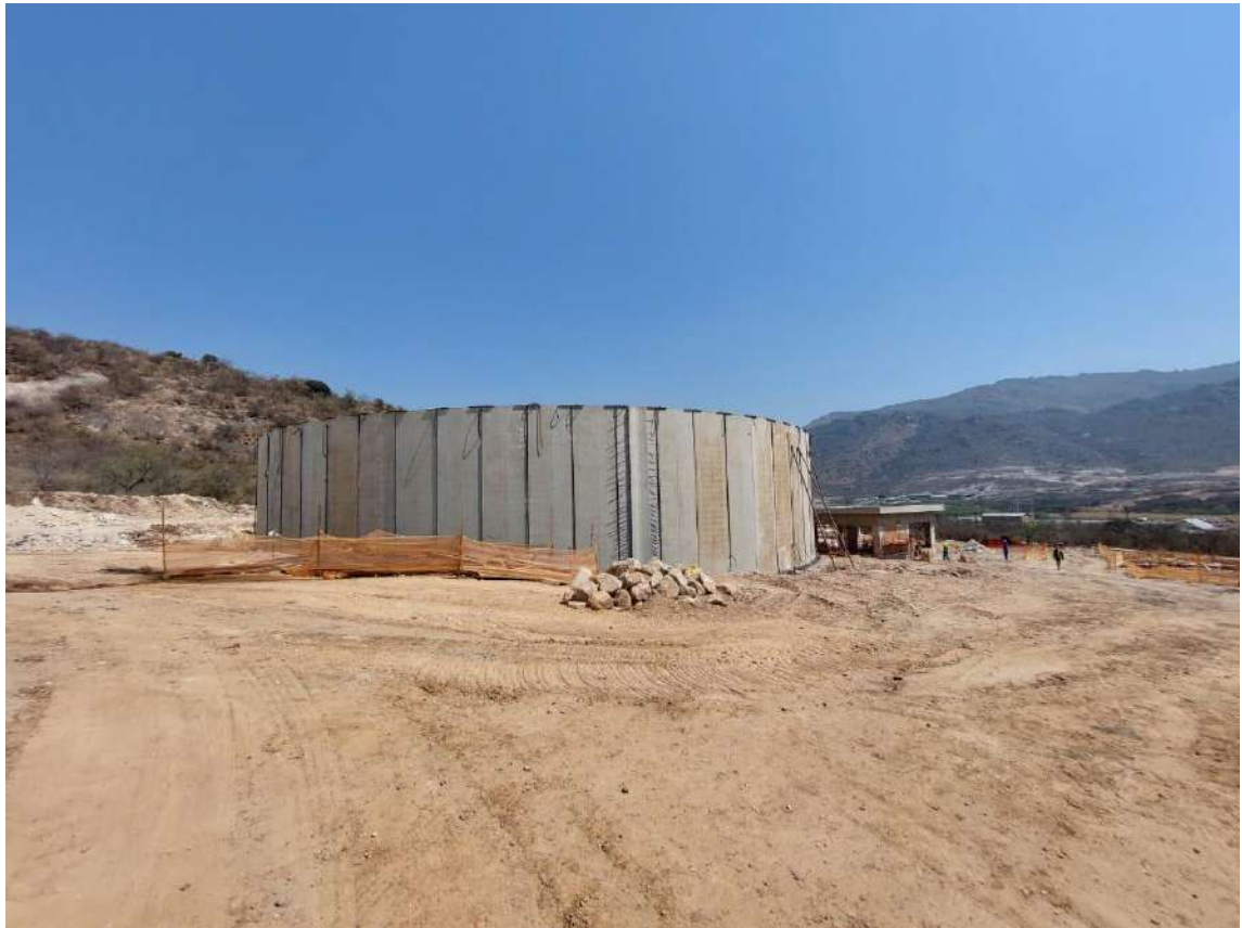
Photo 48: Excavation at Reservoir Site
