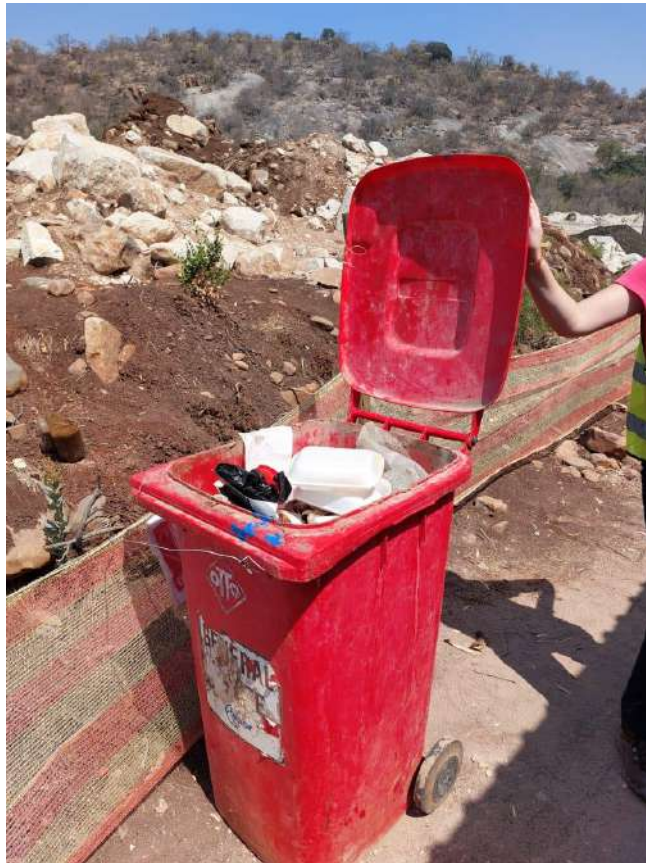
Photo 29: Waste Management at Reservoir site
