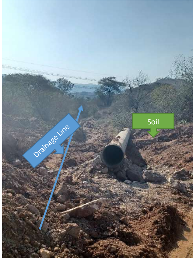
Photo 31: Soil stored in the drainageline and sandbags washed away
