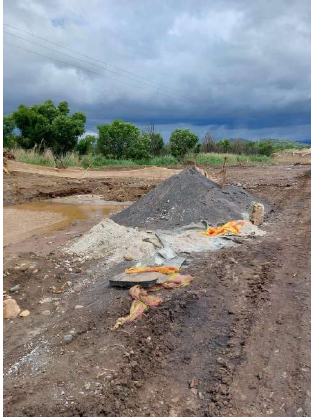
Photo 35: Mixing of concrete taking place within wetland area
