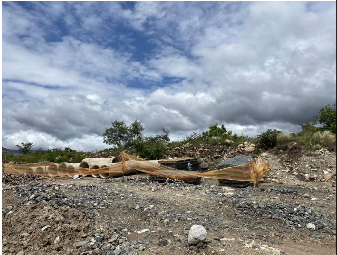
Photo 37: Construction site areas demarcated with reflector netting
