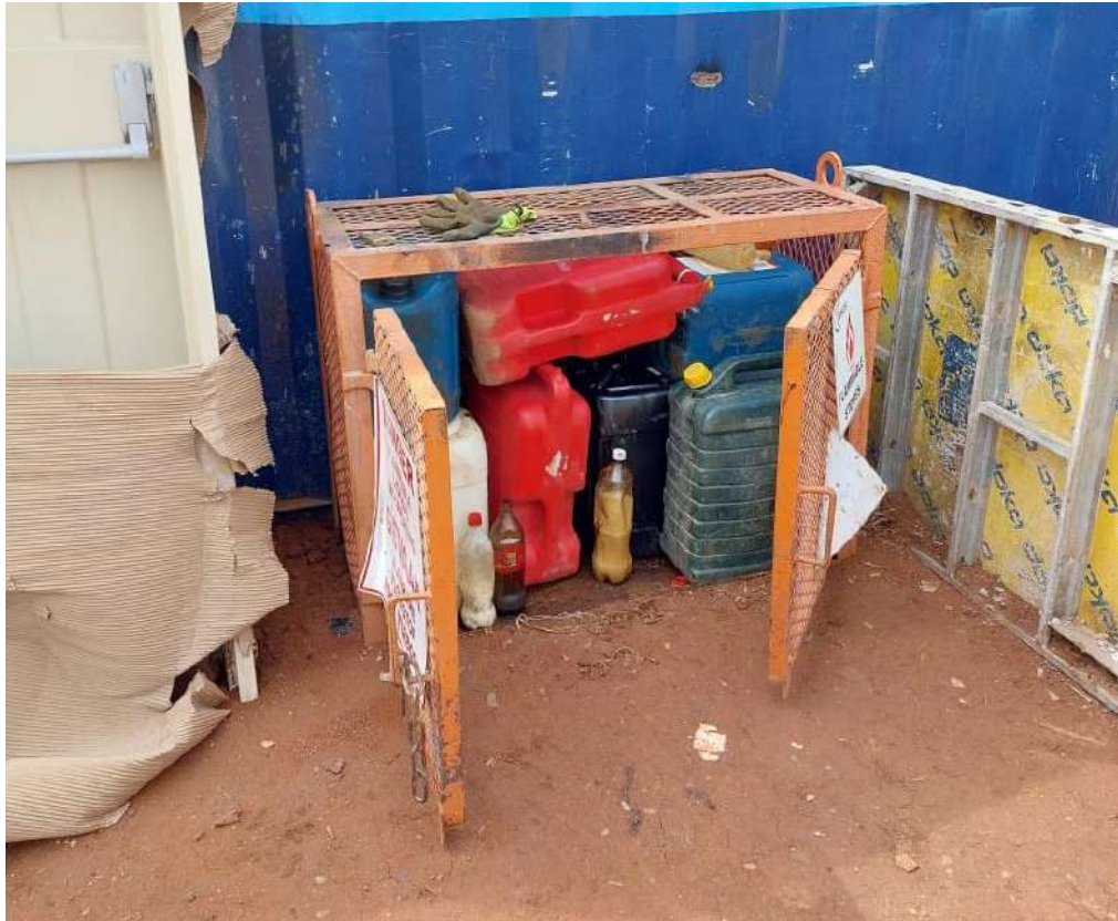
Photo 40: Chemical Storage Cage unlocked
