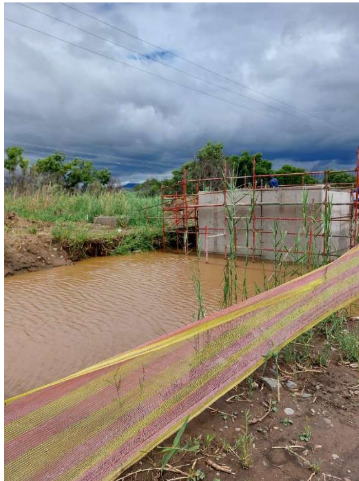
Photo 44: Wetland area – Construction and secondary activities
