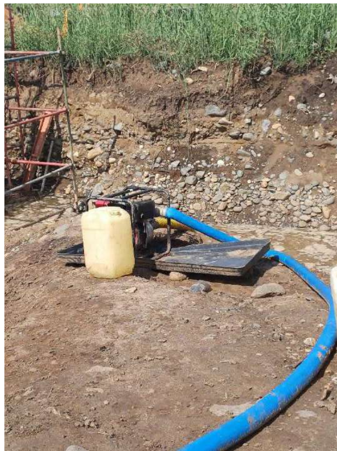
Photo 34: Drip trays found under machinery on site
