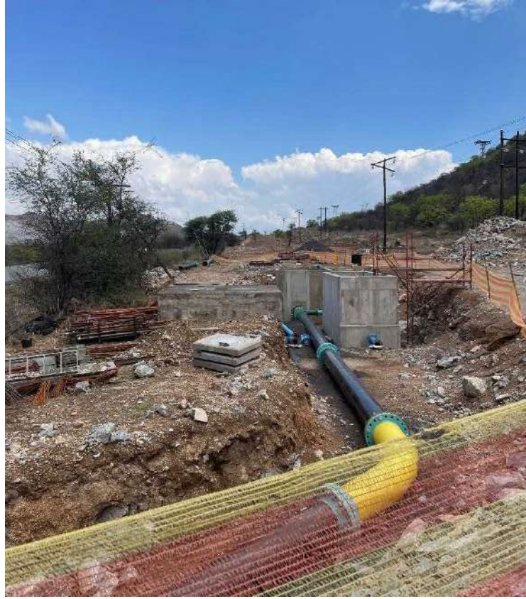
Photo 49: Deep hole excavation at man hole site
