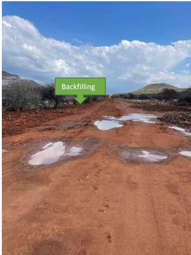
Photo 18: Backfilling of Subsoil on the pipeline route
