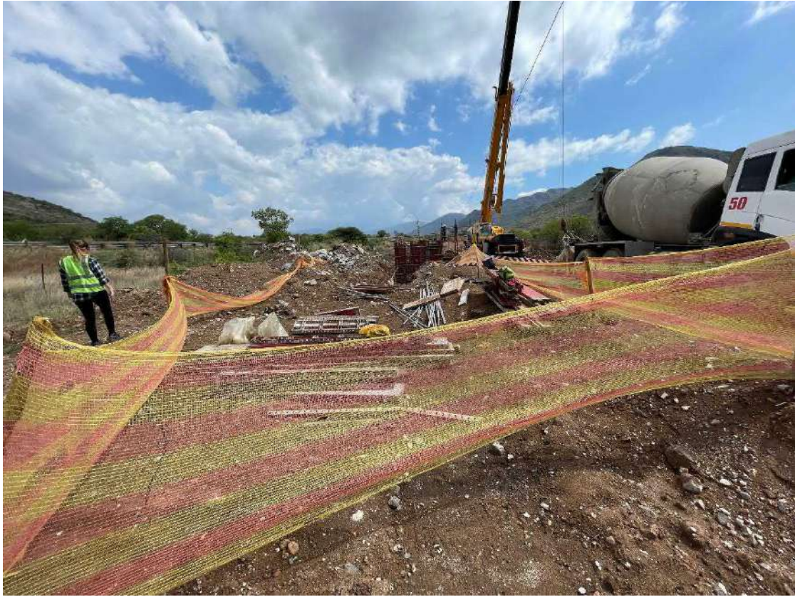
Photo 37: Construction site areas demarcated with reflector netting
