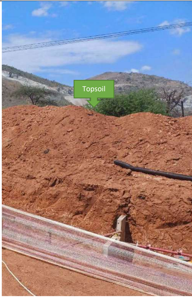
Photo 18: Backfilling of Subsoil on the pipeline route
