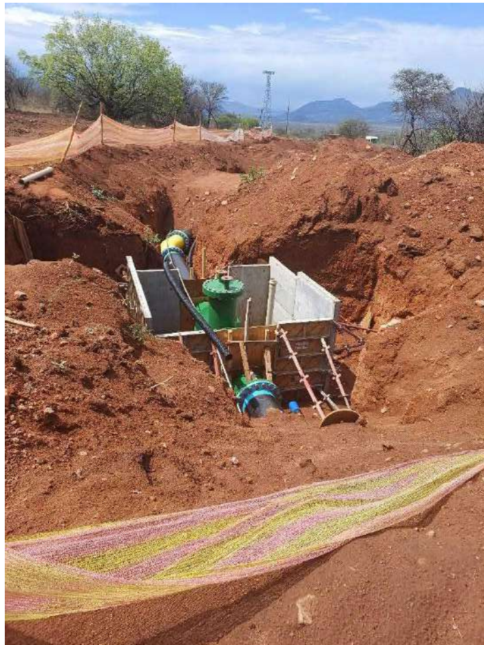
Photo 49: Deep hole excavation at man hole site
