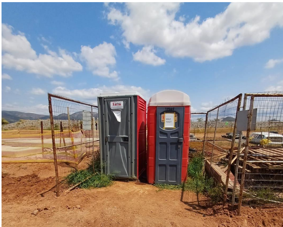
Spitskop Pump Station
