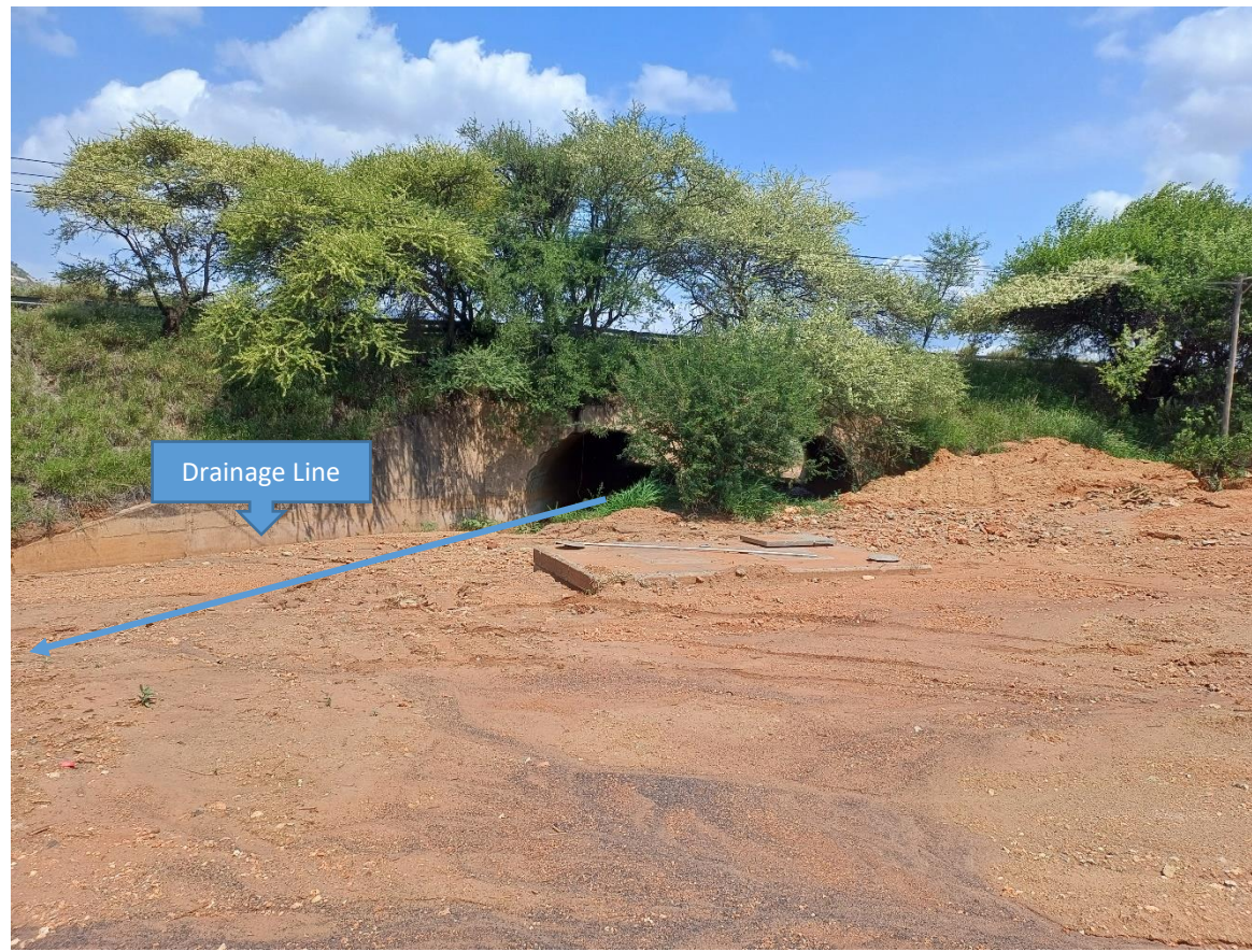
Photo 31: Soil removed from drainageline
