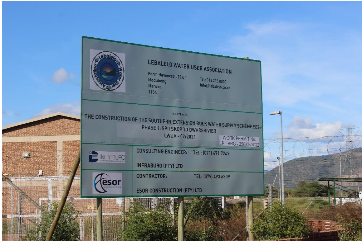
Photo 47: Construction signage on site
