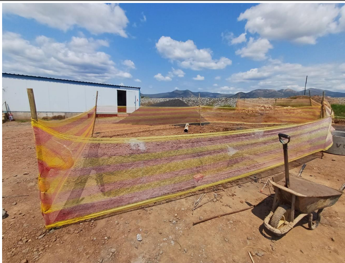
Photo 37: Construction site areas demarcated with reflector netting
