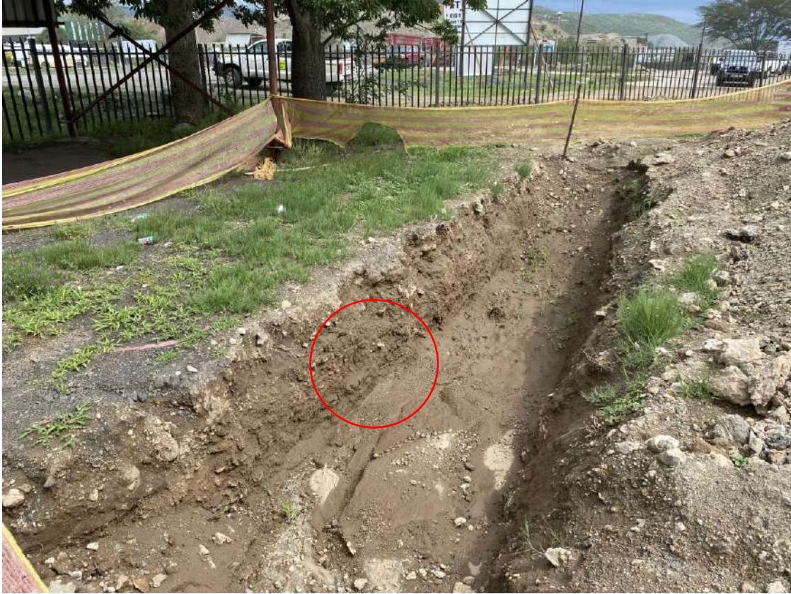
The picture below is from the November 2023 Audit
