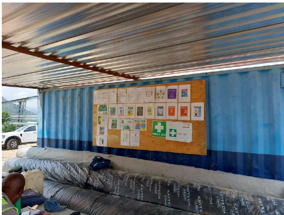
Photo 45: Construction and safety signage on site
