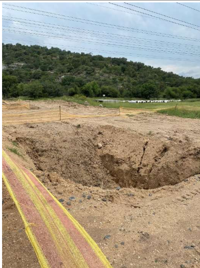
Photo 36: Construction site areas demarcated with reflector netting
