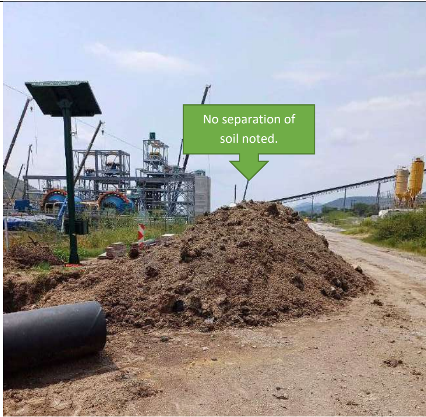
Photo 18: Backfilling of Subsoil on the pipeline route
