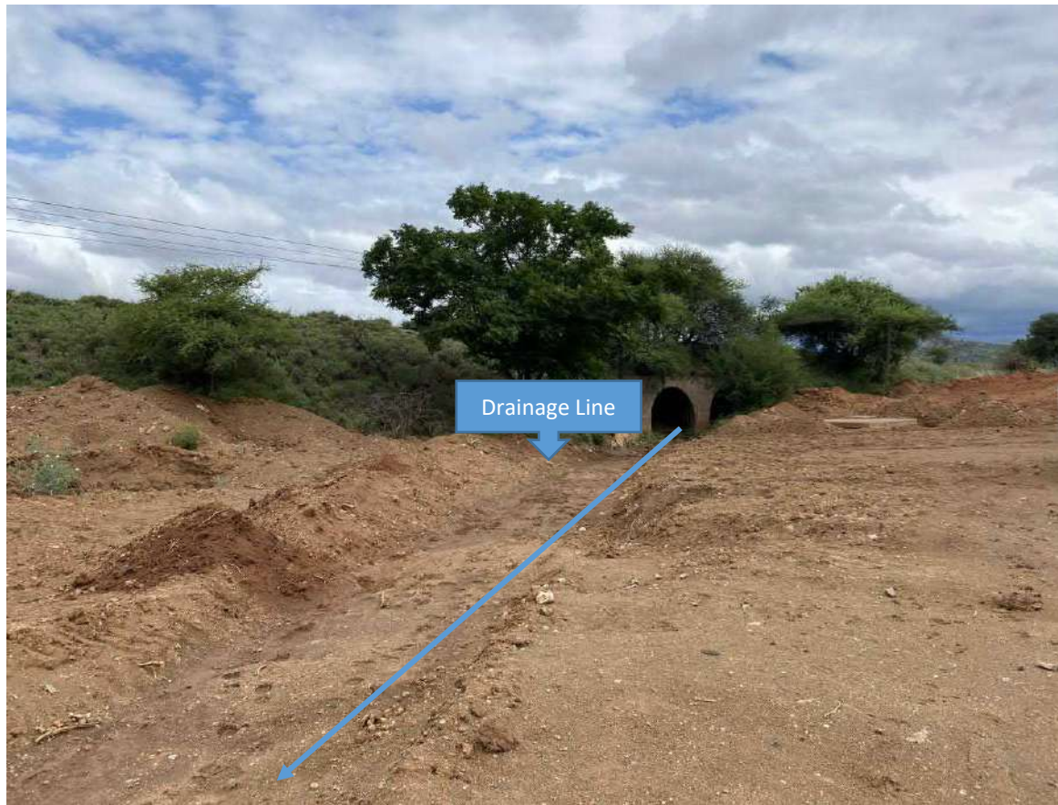
Photo 32: Soil removed from drainageline
