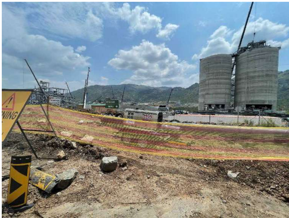
Photo 36: Construction site areas demarcated with reflector netting
