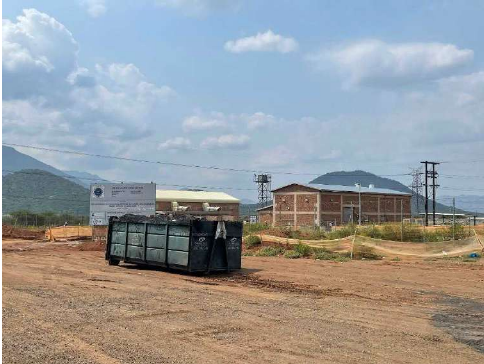
Photo 26: Spitskop Pump Station Waste Management
