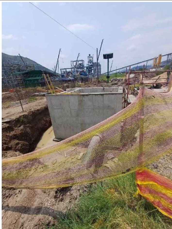
Photo 48: Deep hole excavation at man hole site
