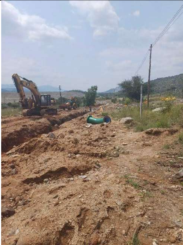
Photo 48: Deep hole excavation at man hole site
