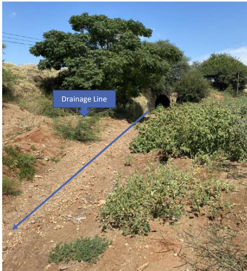
Photo 31: Soil removed from drainageline
