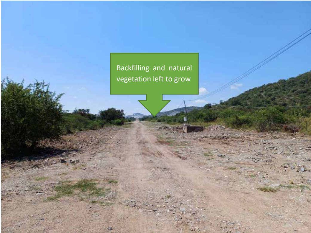
Photo 18: Backfilling of Subsoil on the pipeline route
