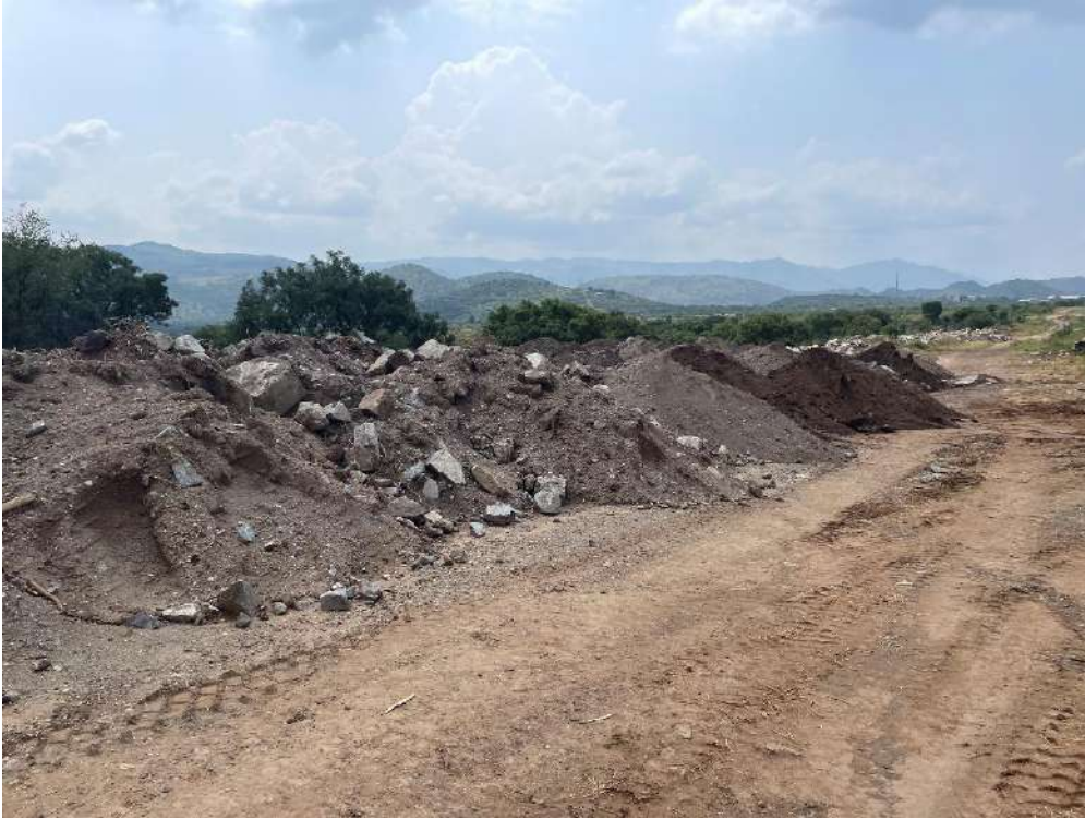
Photo 29: Waste Management along pipeline route
