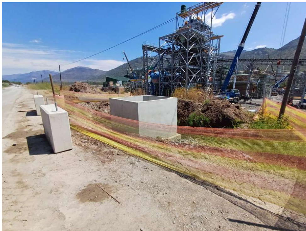
Photo 36: Construction site areas demarcated with reflector netting
