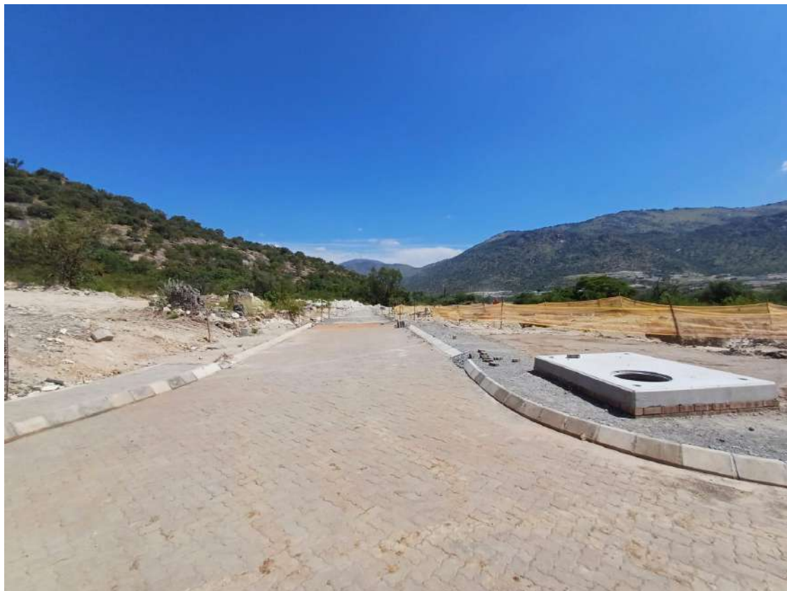
Photo 47: Construction Activities at Dwarsrivier Pump Station
