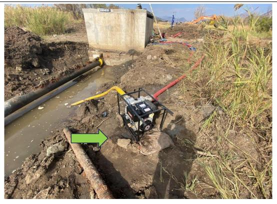
Photo 36: No drip trays being used on site
