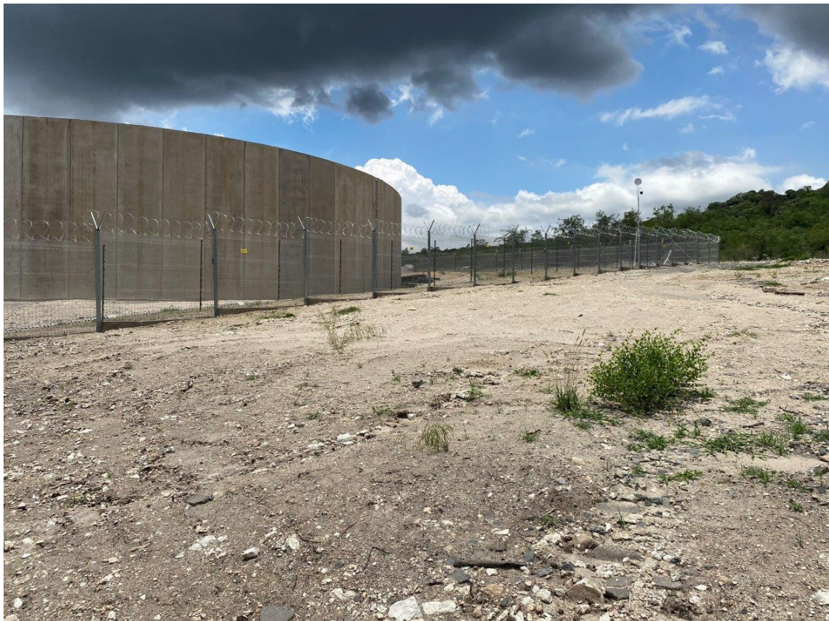
Photo 8: Area at New Reservoir that has not re-vegetated
